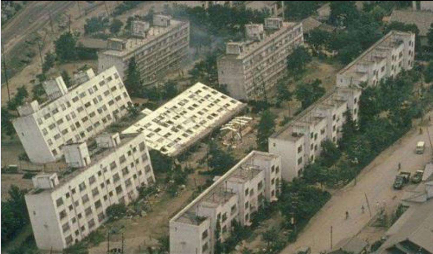
Perdita di portanza (loss of bearing strength)
